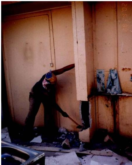
**Figure-7.** Dismantling operations with inappropriate labor tools
